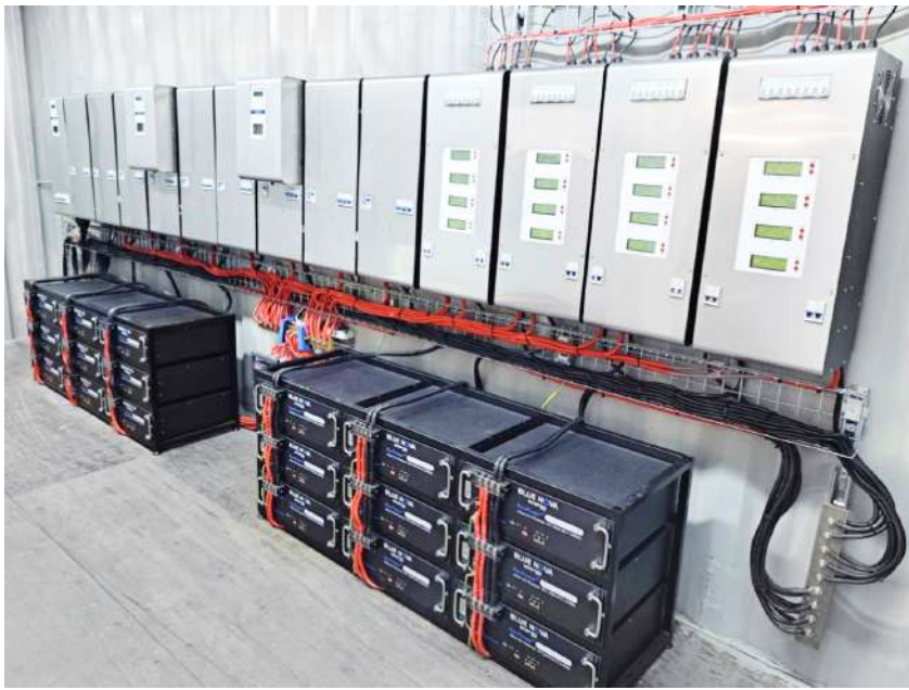
75kW Three-Phase Mini-Grid with 90kW Li-Ion Batteries
