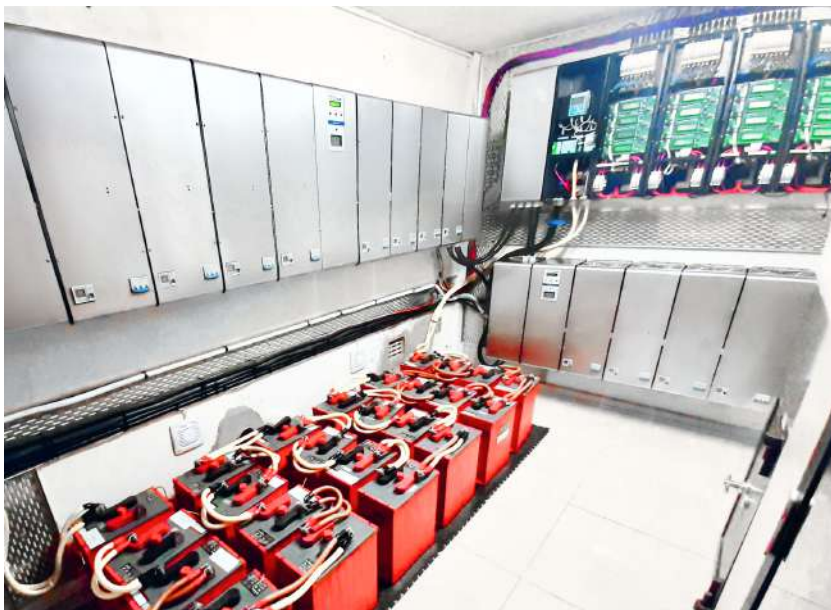
60kW Three-Phase Mini Grid with Intelligent DC Charger
