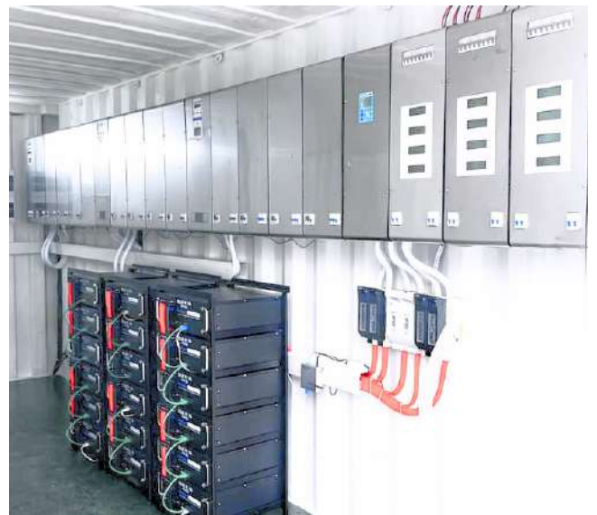
Containerised 60kW Three-Phase Mini-Grid with 30kWp Solar Power
