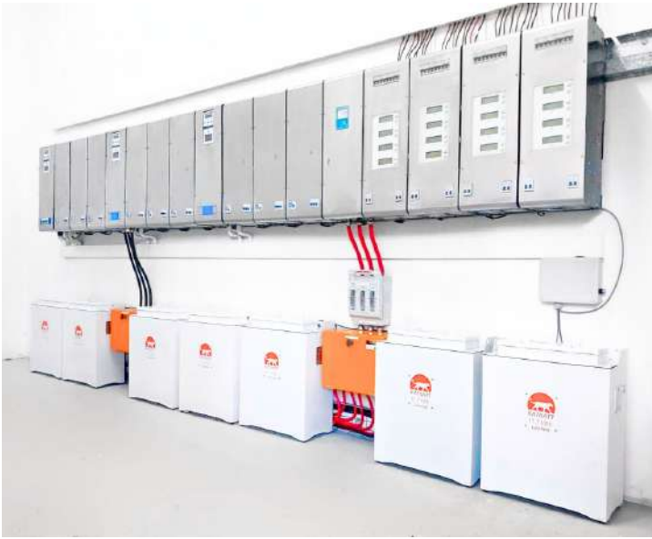
45kW Mini-Grid System
