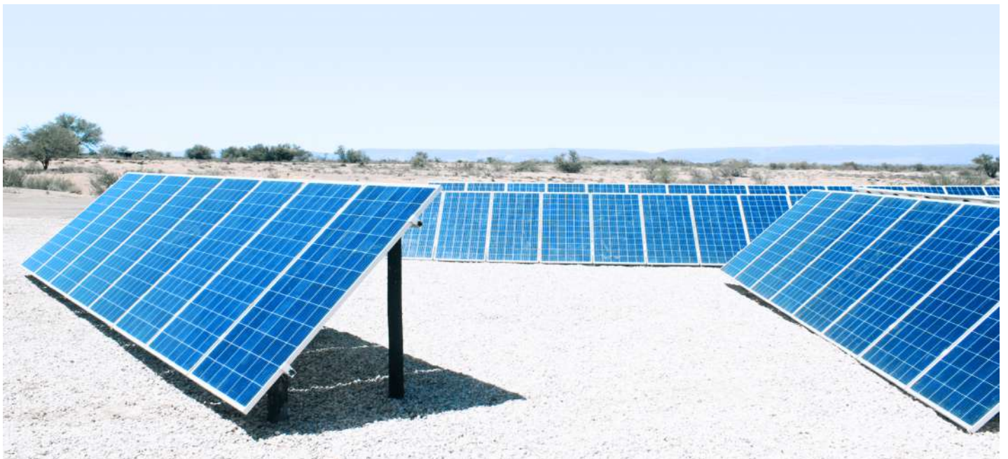
60kW Three-Phase Mini-Grid powering a farm (Ground Mount Solar)
