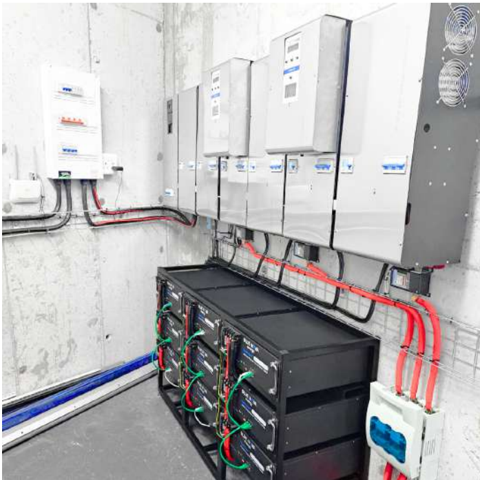
46kWh Li-Ion Battery Bank
