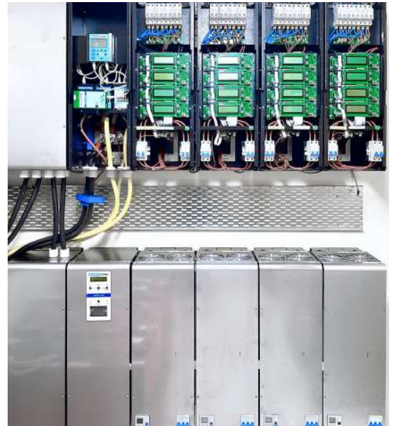
60kW Three-Phase Mini Grid with Intelligent DC Charger
