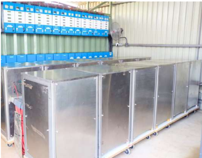
90kW Single-Phase with 864kWh Battery
