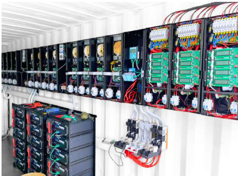
Containerised 60kW Three-Phase Mini-Grid with 30kWp Solar Power
