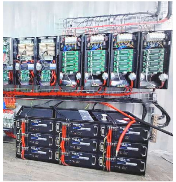
75kW Three-Phase Mini-Grid with 90kW Li-Ion Batteries
