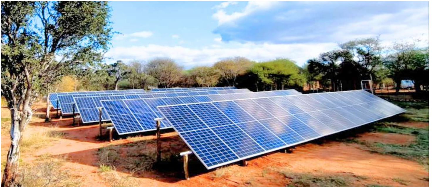
40kW Ground Mount Solar System for the Mini-Grid
